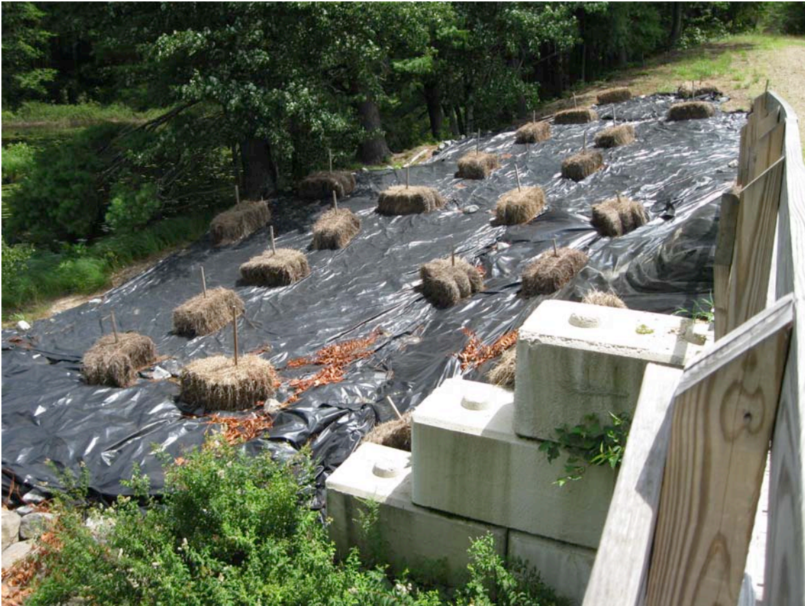
Close-up view of southeast corner of Black Brook bridge embankment. Knotweed infestation was only on the south side of the bridge because fill from highway ditch diggings was used to build up the bridge approach on this side.
